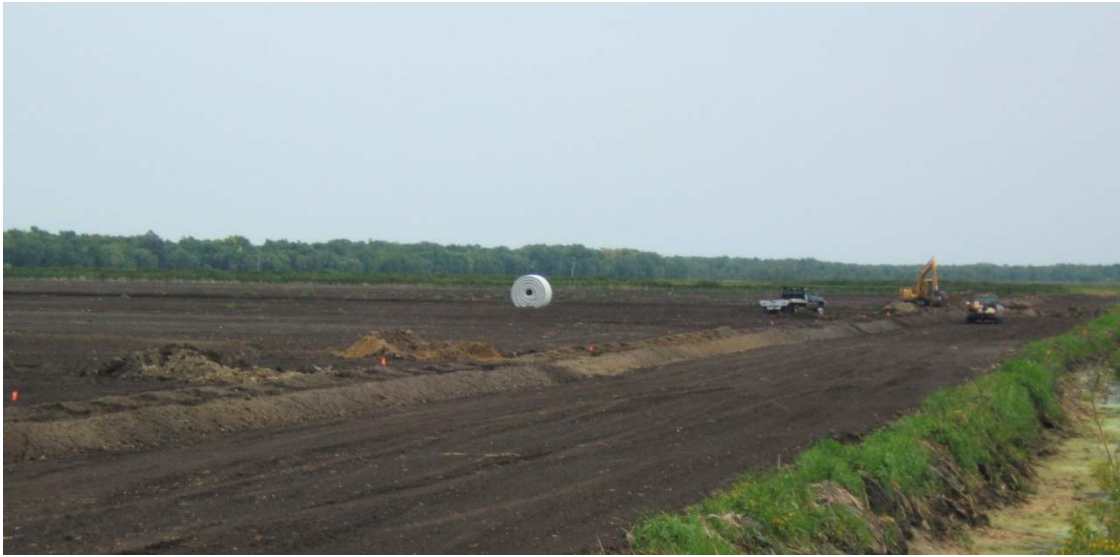
Figure 2. Installation of wild rice paddy tile drainage
